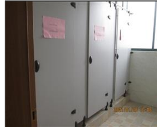
Photo of the sanitary facilities Toilet.JPG
