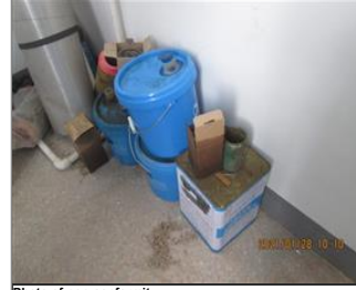
Photo of non-conformity NC No secondary containment and no MSDS and no safety labels.JPG
